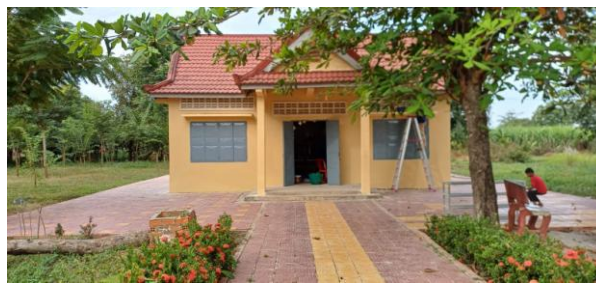
Library after refurbishment
